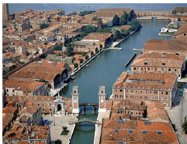
Figure 3 . The Arsenale Vecchio shipyard dock basin experiment area
