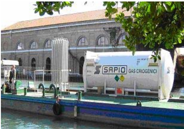
Figure 4 . The 20 000 liter cryogenic evaporator
